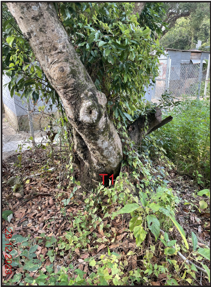
T1 Ground Condition
